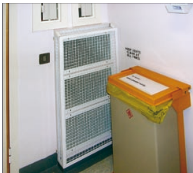
Pressure stabiliser with stand-off cage
